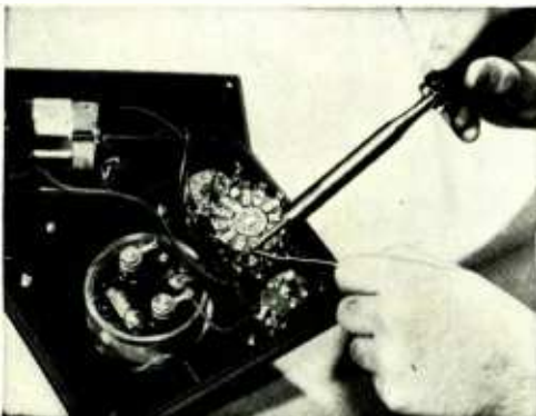
Construction of Multimeter.
